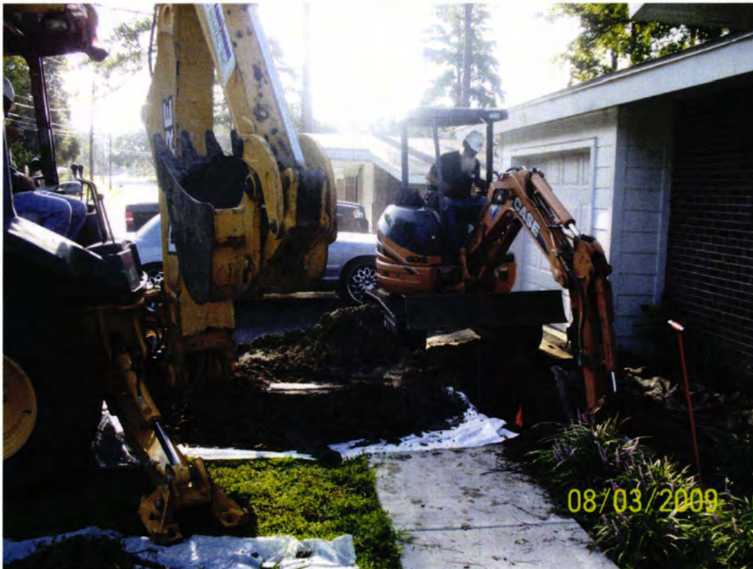
Picture 2: Extraction of UST at 1426 Albatross.
